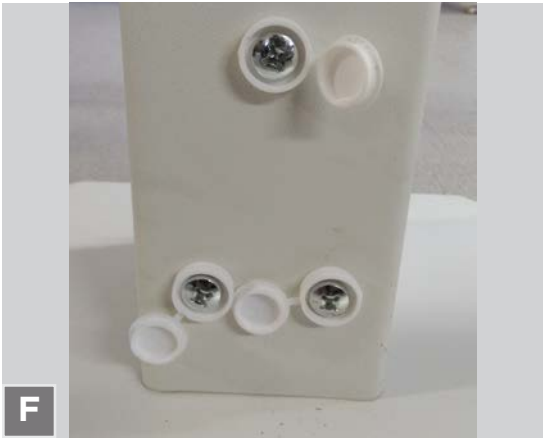
Power pole back screw and covers installed
