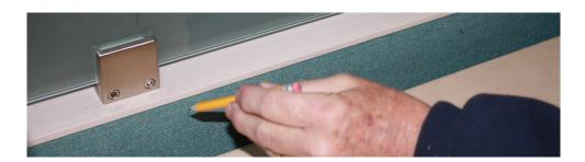
2. Panel does not have the holes drilled upon arrival. To start, put PGHM on mullion and then hold in place on the panel.
