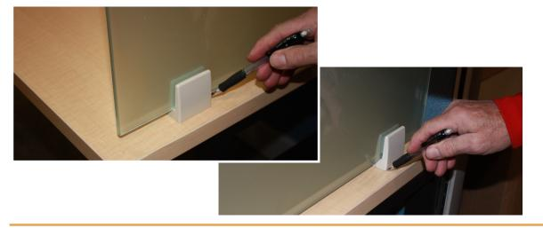
2. Worksurface does not have the holes drilled upon arrival. To start, put PGHM on mullion and then hold in place on the worksurface.
