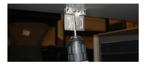
6. Establish your hole location. Mount the block using 2 1" Phillips screws.
