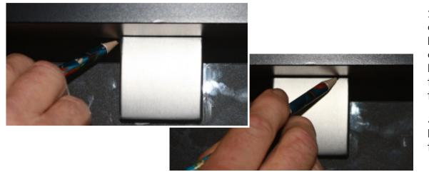
2. Worksurface/Panel does not have the holes drilled upon arrival. To start, put PGHM on mullion and then hold in place on the worksurface.
